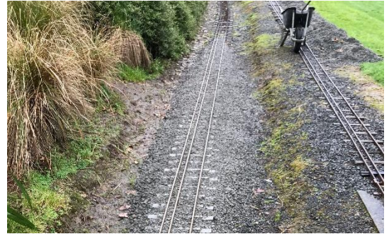
A layer of ballast added to some new track on the climb towards the back of the Outside Track.
