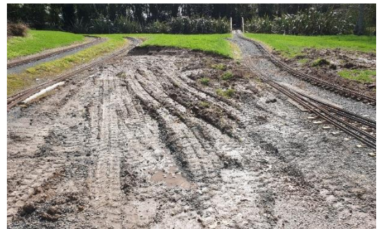
The first section of dirt dug out in preparation for laying new track.
