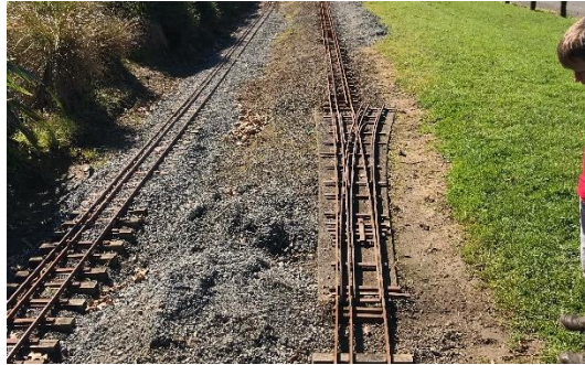
A new point installed on the branch line to the steaming bays, ready for the additional loop.
