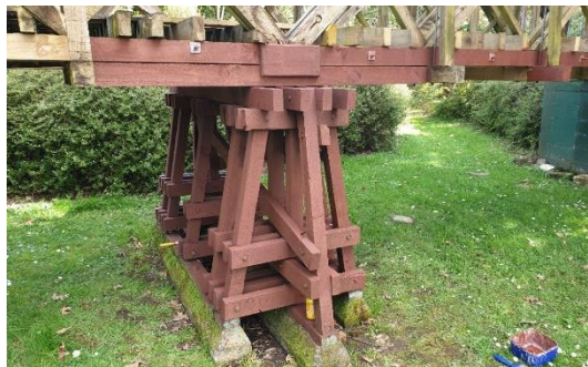
The first layer of paint going over the repaired trestle bridge. Looks great!
