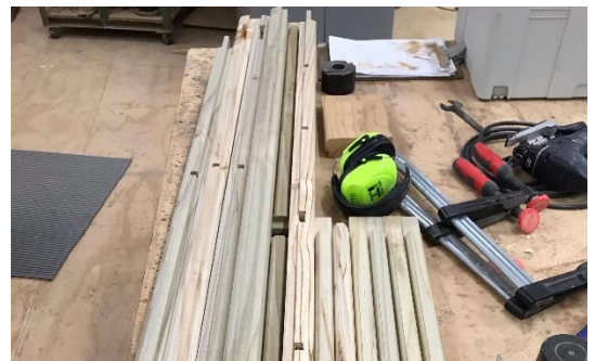
All pieces of the new sash ready to go together like a lifesize set of lego!
